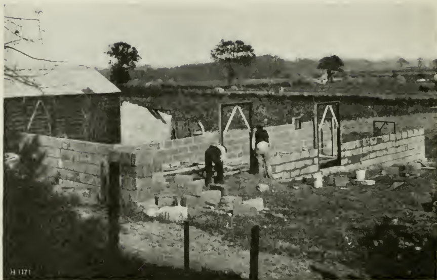
FIG. 70.—A FARM BUILDING IN COURSE OF CONSTRUCTION.
